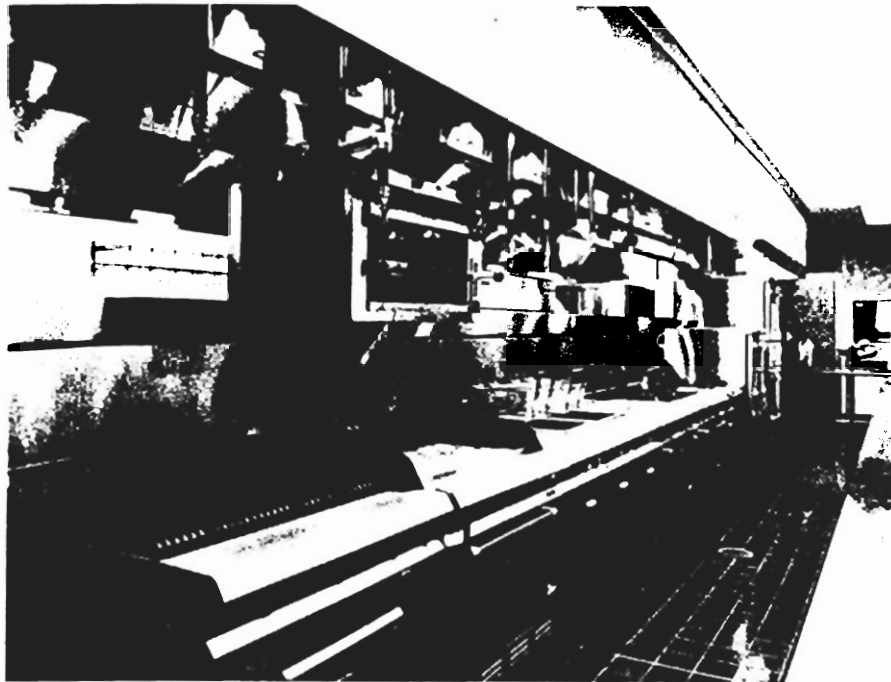
Shown here: a typical hood with the Gaylord Quencher™ Water Spray Fire Protection System. Pre-engineered for commercial kitchen cooking appliances and exhaust systems. For use in buildings with a sprinkler system, it is installed by the fire sprinkler contractor. System utilizes Grinnell's Model EA-1 nozzles.
